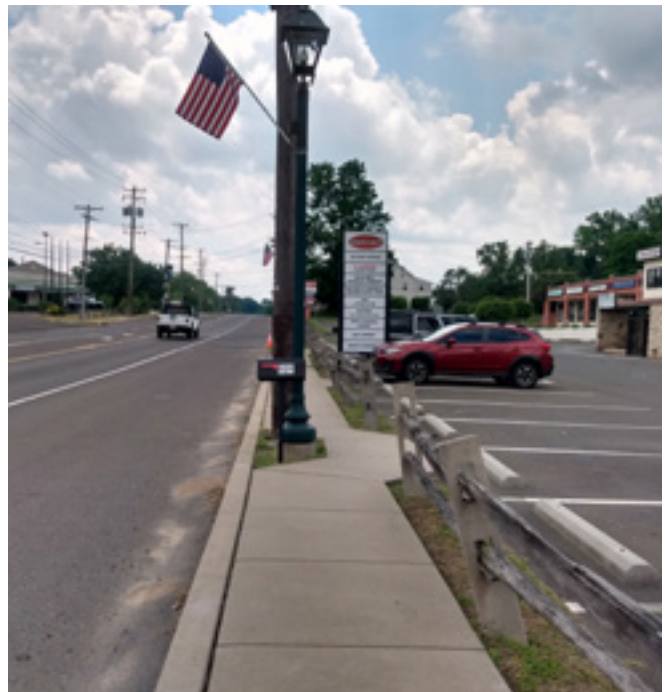
A narrow sidewalk and lack of buffer between the road and sidewalk create an unfriendly pedestrian environment.
