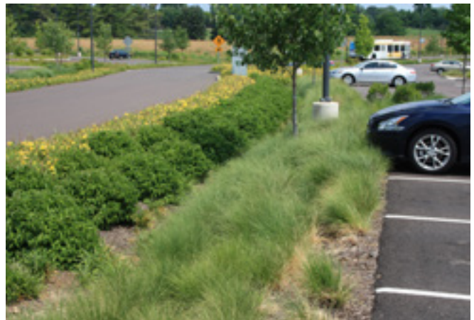
Parking lot infiltration.
