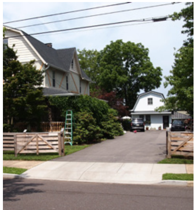
Detached garage in North Wales, converted to accessory dwelling unit.
