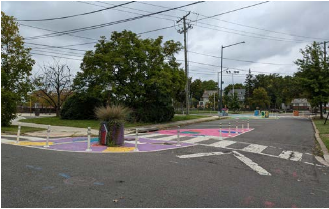
A painted curb extension shortens the street crossing.
