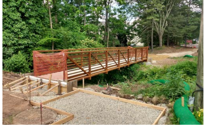
New Bethlehem Pike sidewalks and pedestrian bridge, under construction, summer 2024
