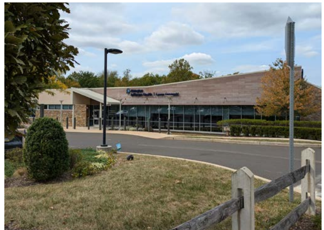
Jefferson Health – Lower Gwynedd, located on Bethlehem Pike.
