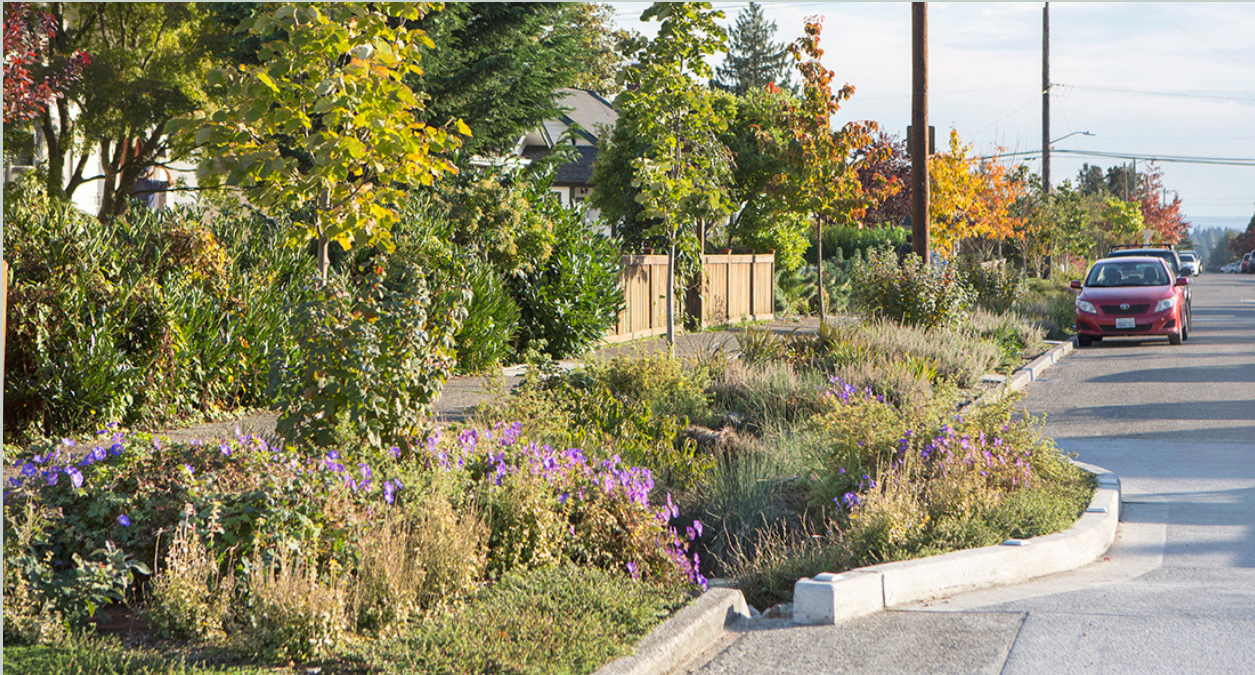
A landscaped bio-retention buffer could be included as part of the space between the sidewalk and the street, sometimes referred to as a verge. As part of the access management study, there should be an analysis of the potential locations for additional greenery along the Bethlehem Pike corridor.
