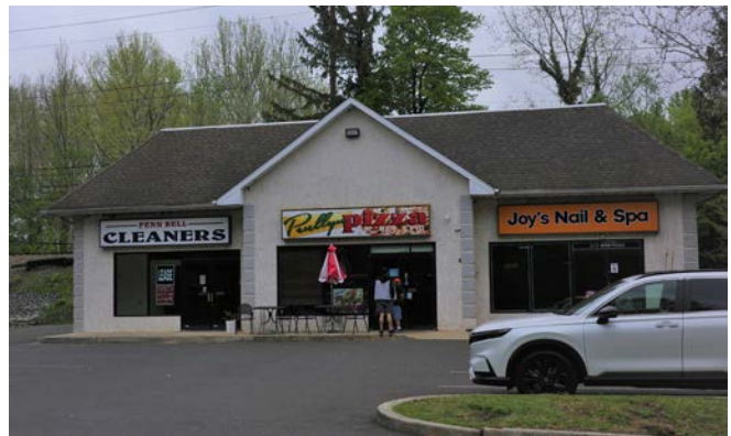
Small-scale commercial near the Penllyn Station
