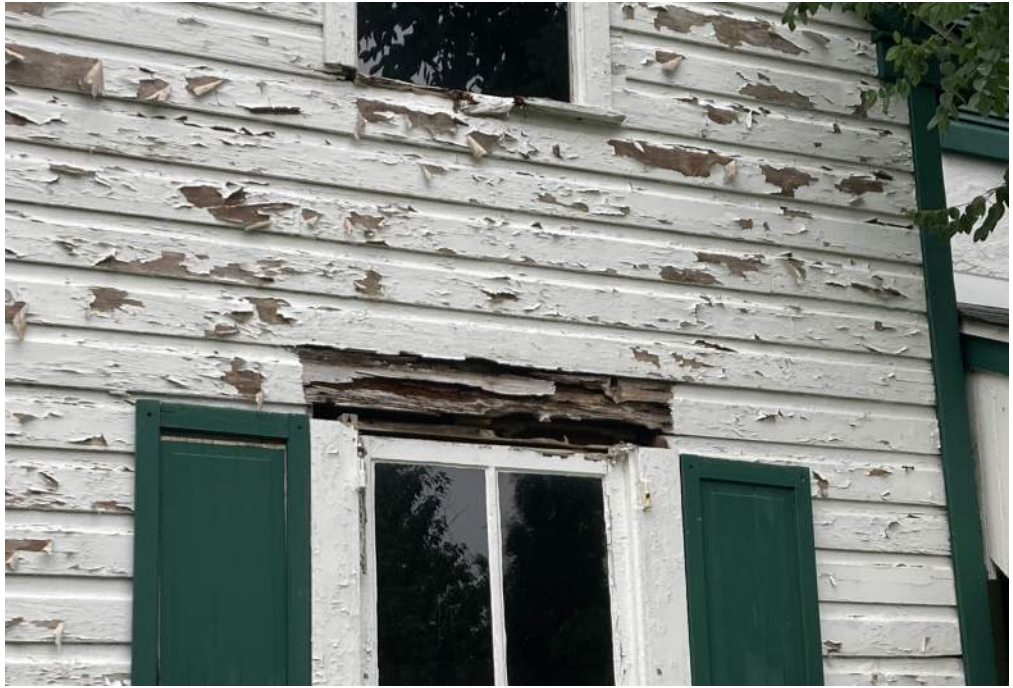
PHOTO 4 DETERIORATED WINDOW HEADER
