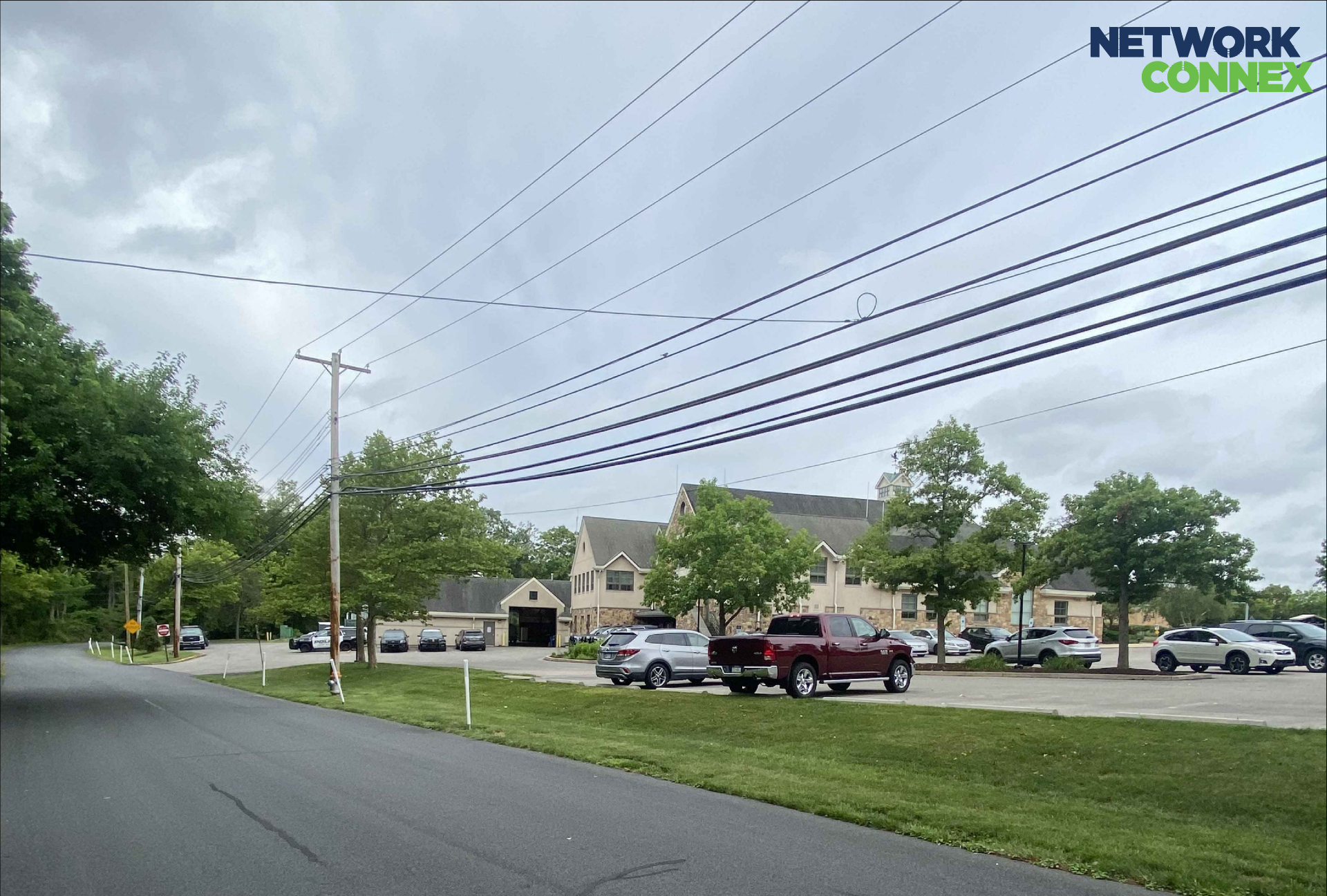
SITE NAME: LOWER GWYNEDD - N. BETHLEHEM (RISE UP) VIEW 1 EXISTING CONDITIONS
