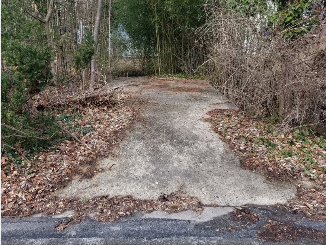
SLAB BRIDGE 448 MARION AVE.
