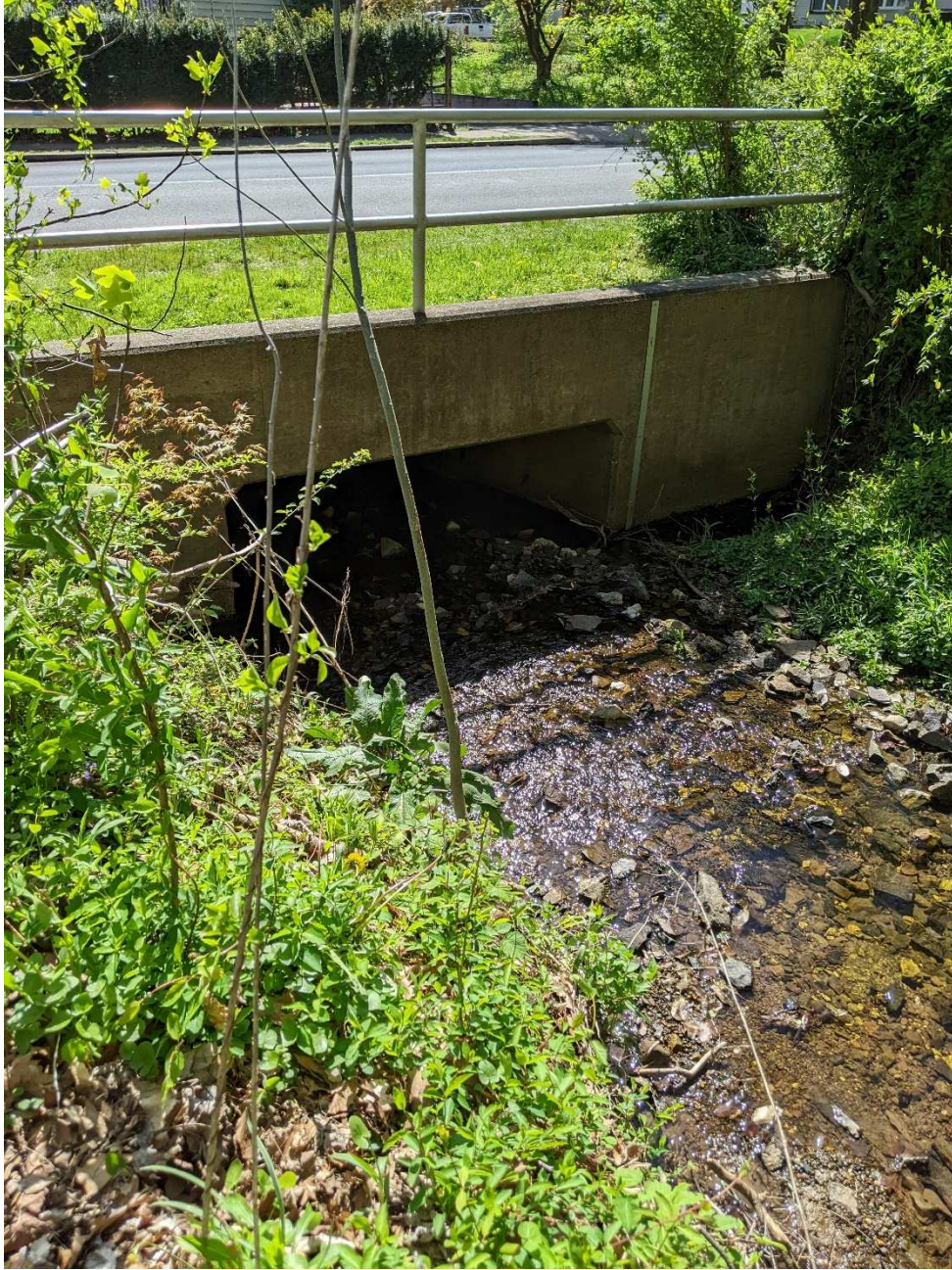
Knight Road Culvert - Upstream
