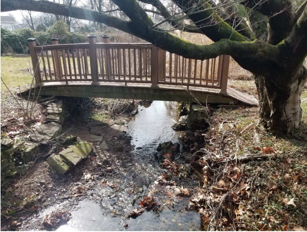
PED BRIDGE 450 MARION AVE.
