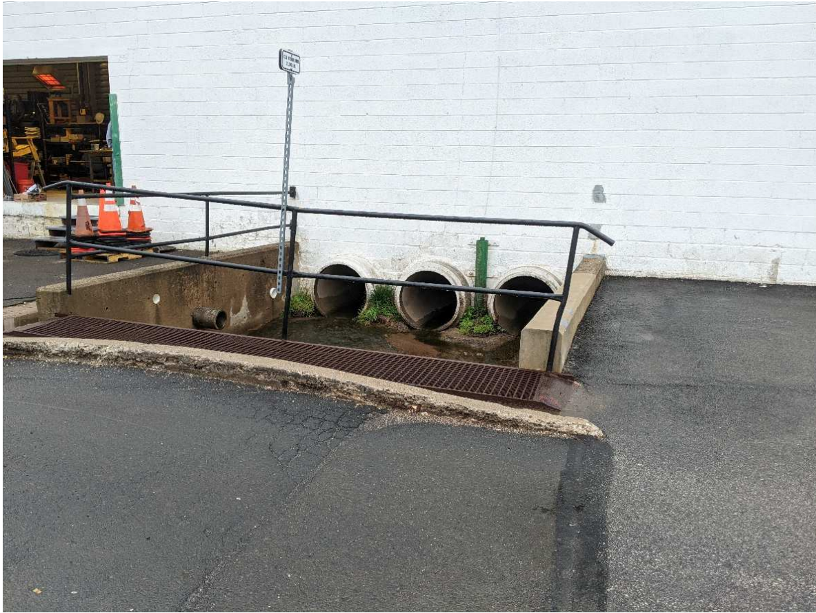
36" PIPES UNDER BUILDING 19 @ AMBLER YARDS
