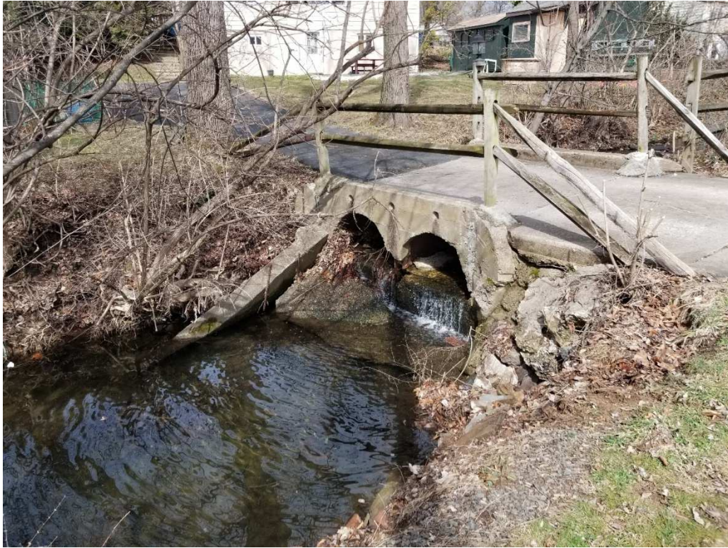
DRIVEWAY BRIDGE 446 MARION AVE.
