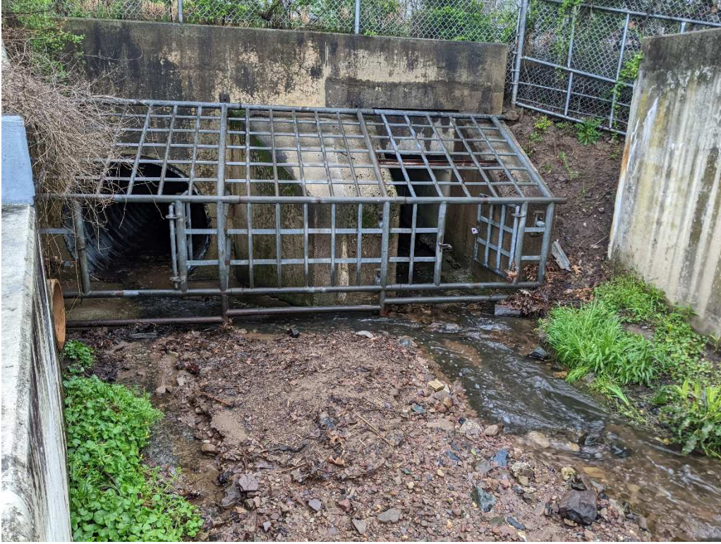
SEPTA CULVERT @ AMBLER YARDS
