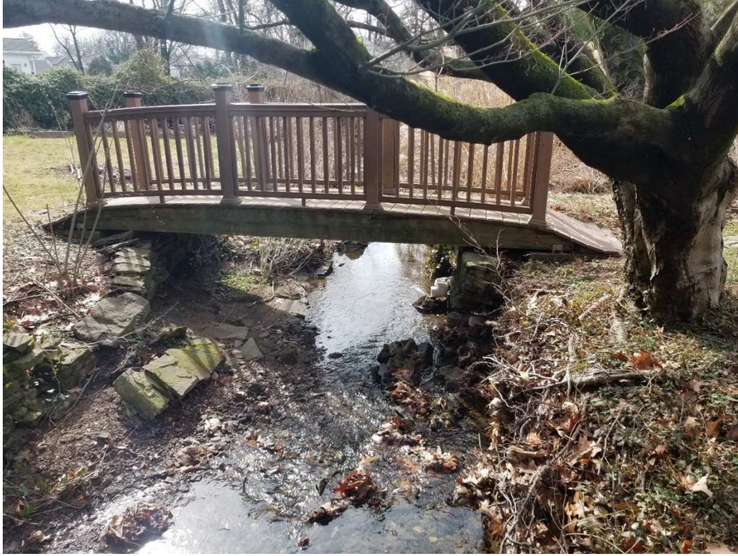
PED BRIDGE 450 MARION AVE.
