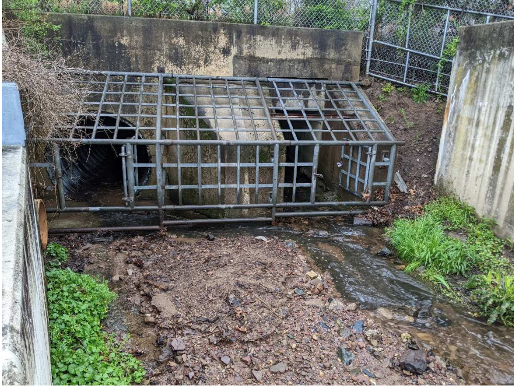
SEPTA CULVERT @ AMBLER YARDS
