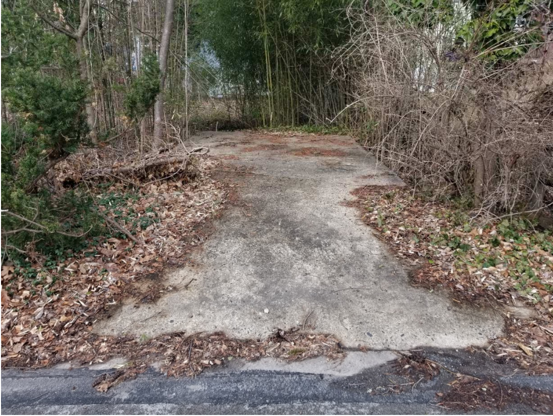
SLAB BRIDGE 448 MARION AVE.
