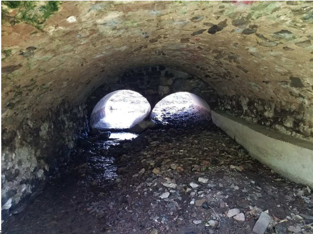
Spring Garden – Culvert (2) 68" x 42" Elliptical Pipes transition to 8' x 4' Box Culvert
