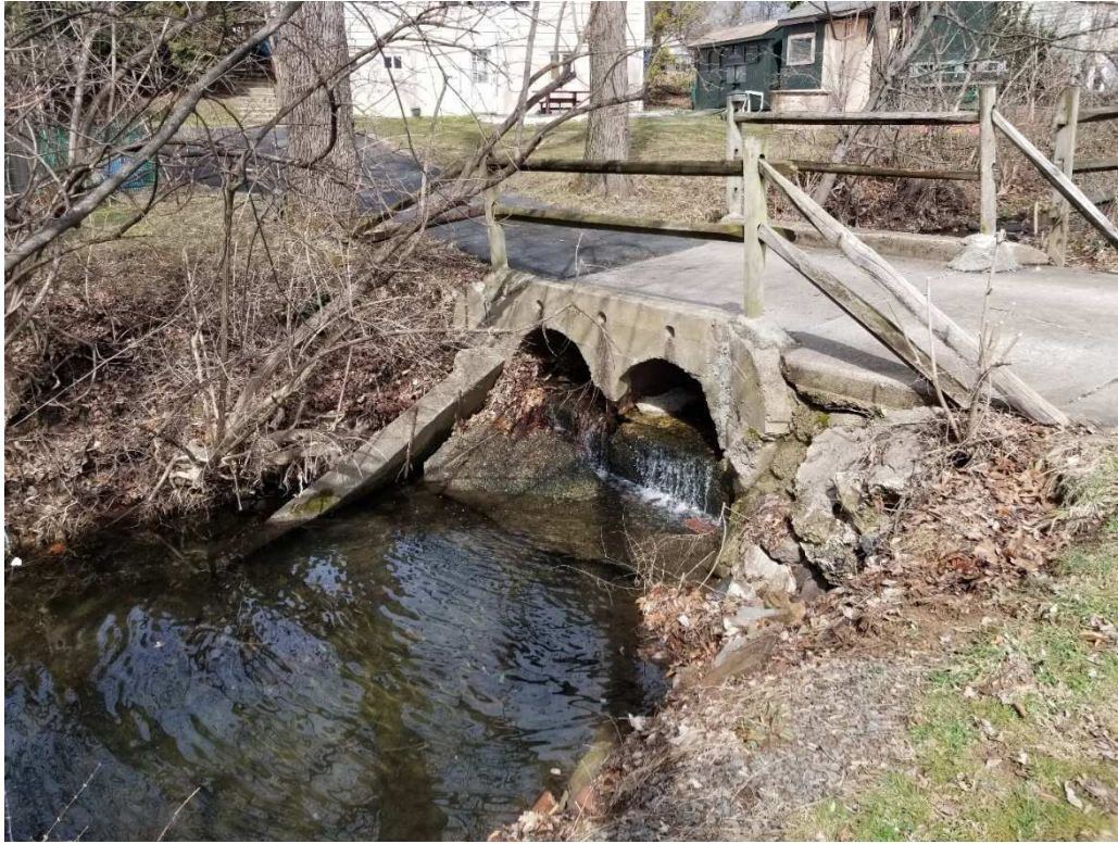
DRIVEWAY BRIDGE 446 MARION AVE.
