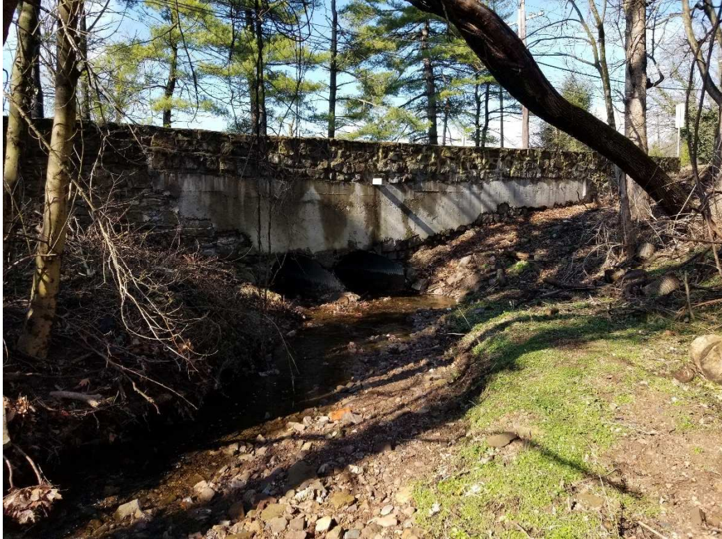
Spring Garden – Culvert (2) 68" x 42" Elliptical Pipes transition to 8' x 4' Box Culvert
