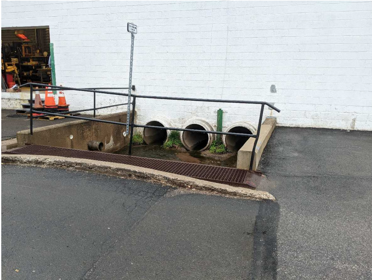
36" PIPES UNDER BUILDING 19 @ AMBLER YARDS
