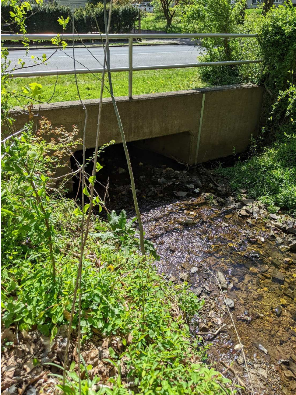
Knight Road Culvert - Upstream
