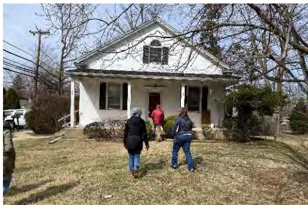
Option C – Consider Renovating the McCormick House to Include Public, Accessible Restrooms
