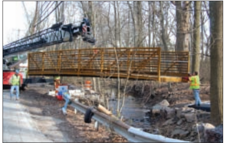
Recent bridge installation for Penlllyn Trail over Penlllyn Creek.
